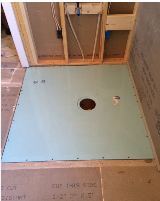
Classic shower base installed on joists.
